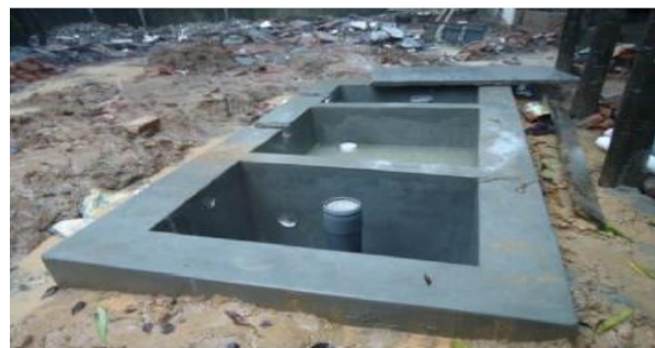
Figure 7: Recharge Well of RWHS (VERC)
